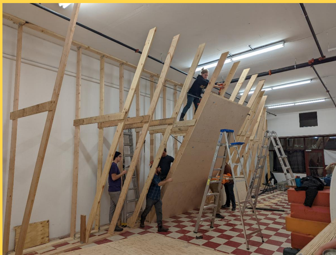
A mix of board members and volunteers work together to hang the first panels on the 30 degree wall
